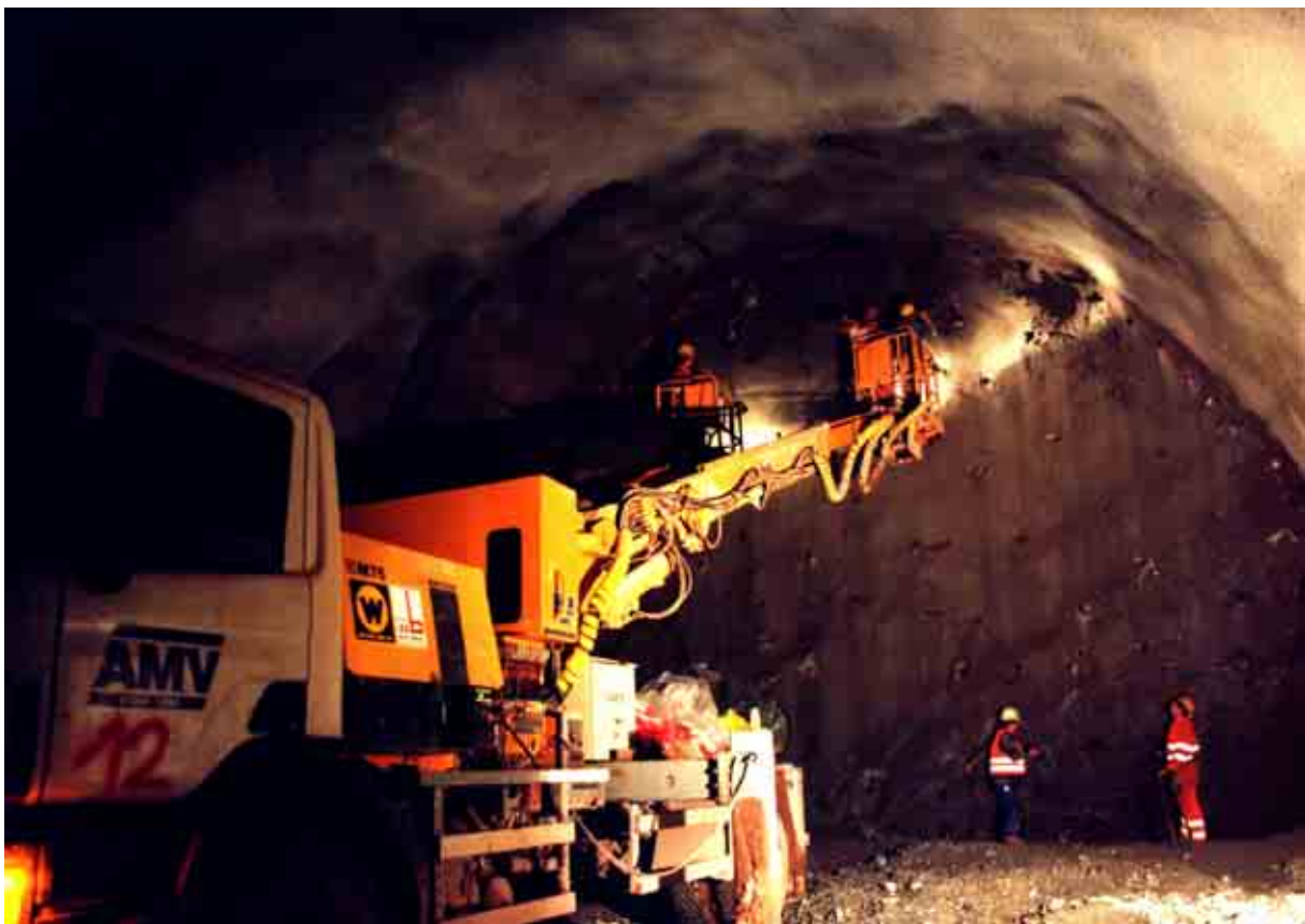
Fig. 6.32: Loading of blastholes during the full-face excavation in granite
