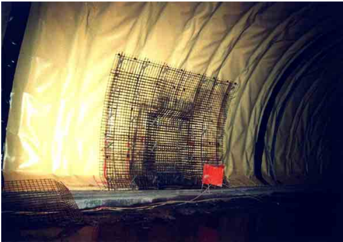
Fig. 6.47: Not reinforced interior lining, reinforcement in the area of a niche
