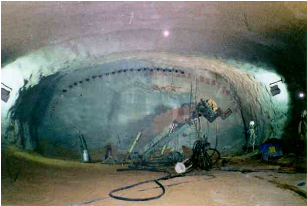
Fig. 4.46: Construction of a pipe umbrella
