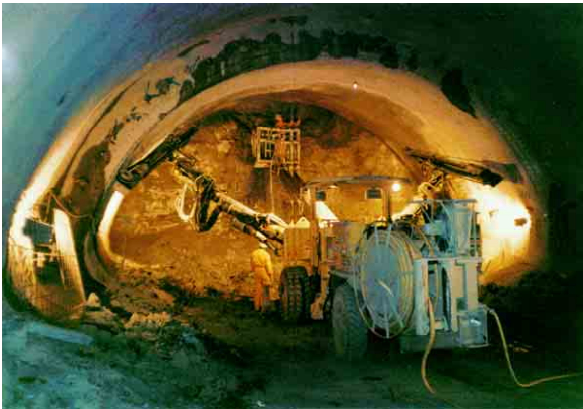
Fig. 4.14: Crown excavation under a pipe umbrella
