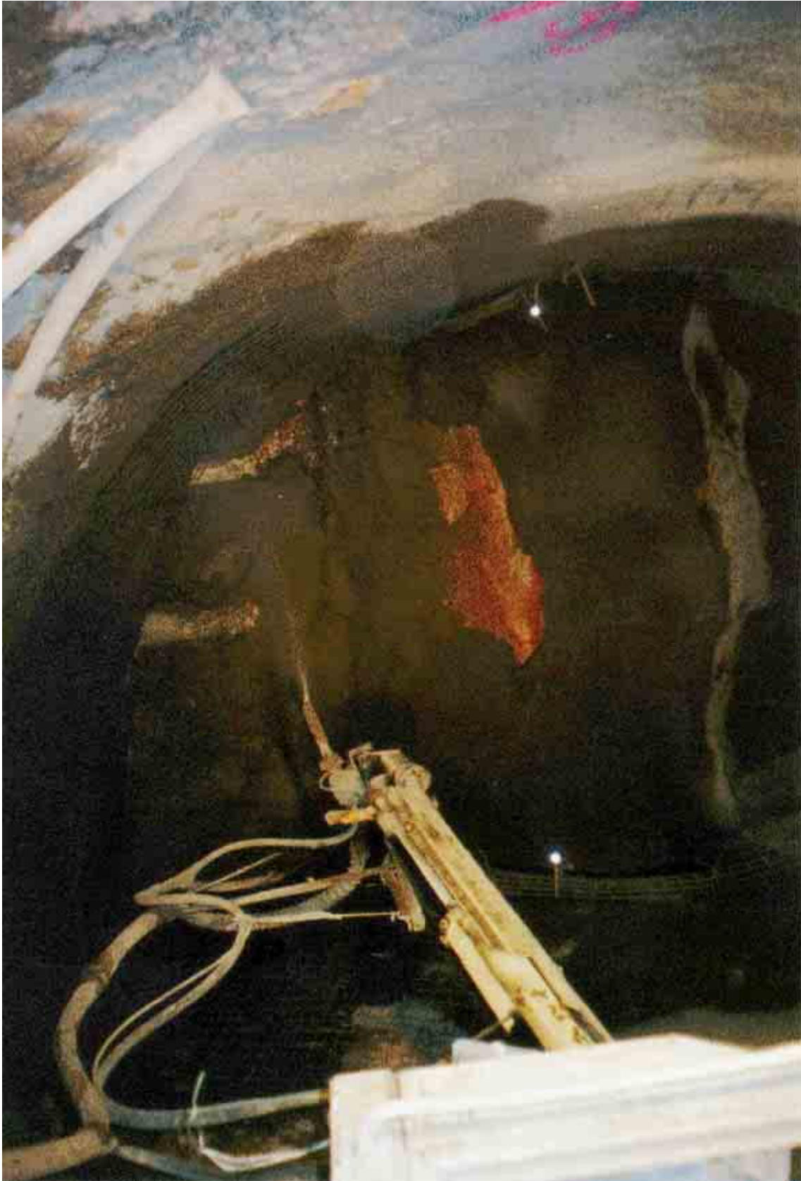
Fig. 2.2: Placing of the shotcrete using a spray vehicle with a remote-controlled spray arm (Limburg Tunnel, new railway line Cologne - Rhine/Main)
