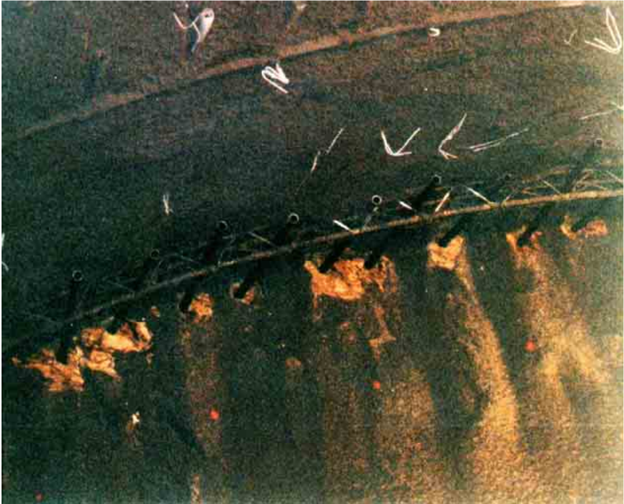
Fig. 2.28: Driven steel pipe spiles (Tunnel Deesener Wald, new railway line Cologne - Rhine/Main)
