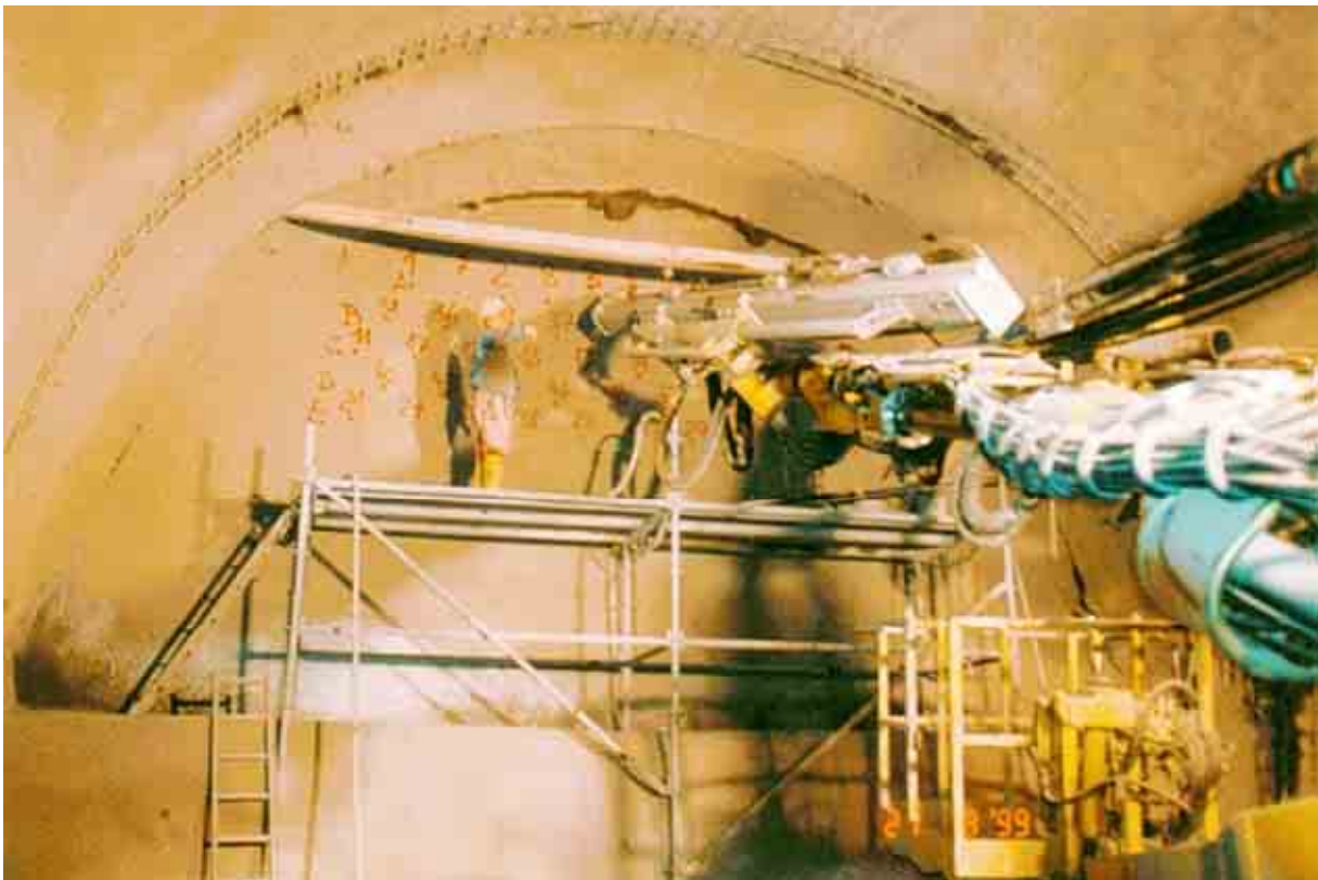
Fig. 6.12: Drilling of grouting boreholes
