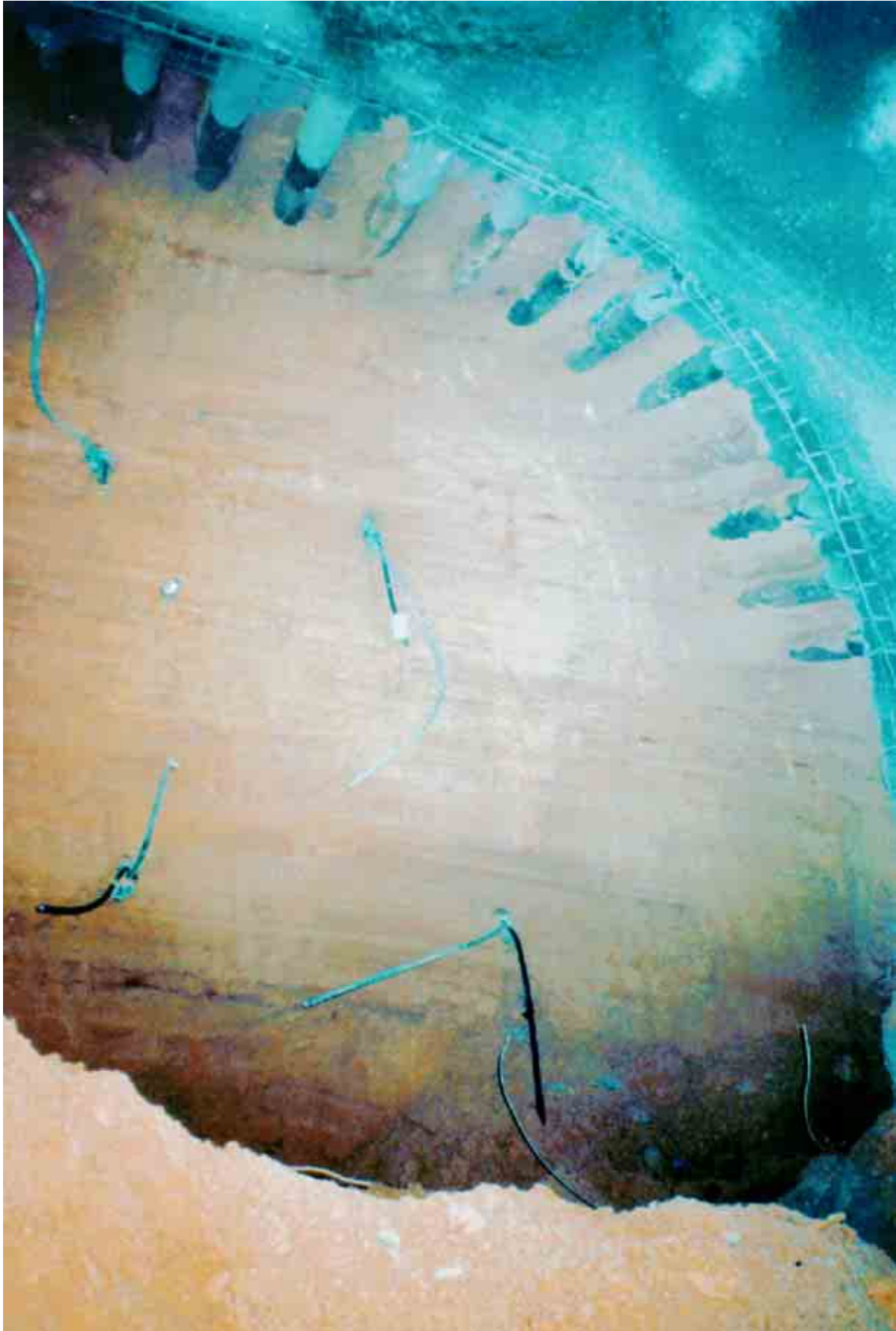
Fig. 4.22: View of the temporary tunnel face located in the "Kurkar" formation
