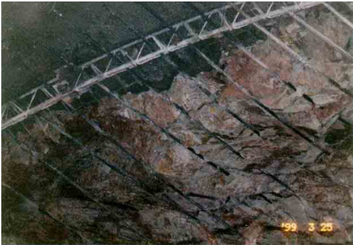
Fig. 2.15: 3-stringer lattice girder (Dernbach Tunnel, new railway line Cologne - Rhine/Main)
