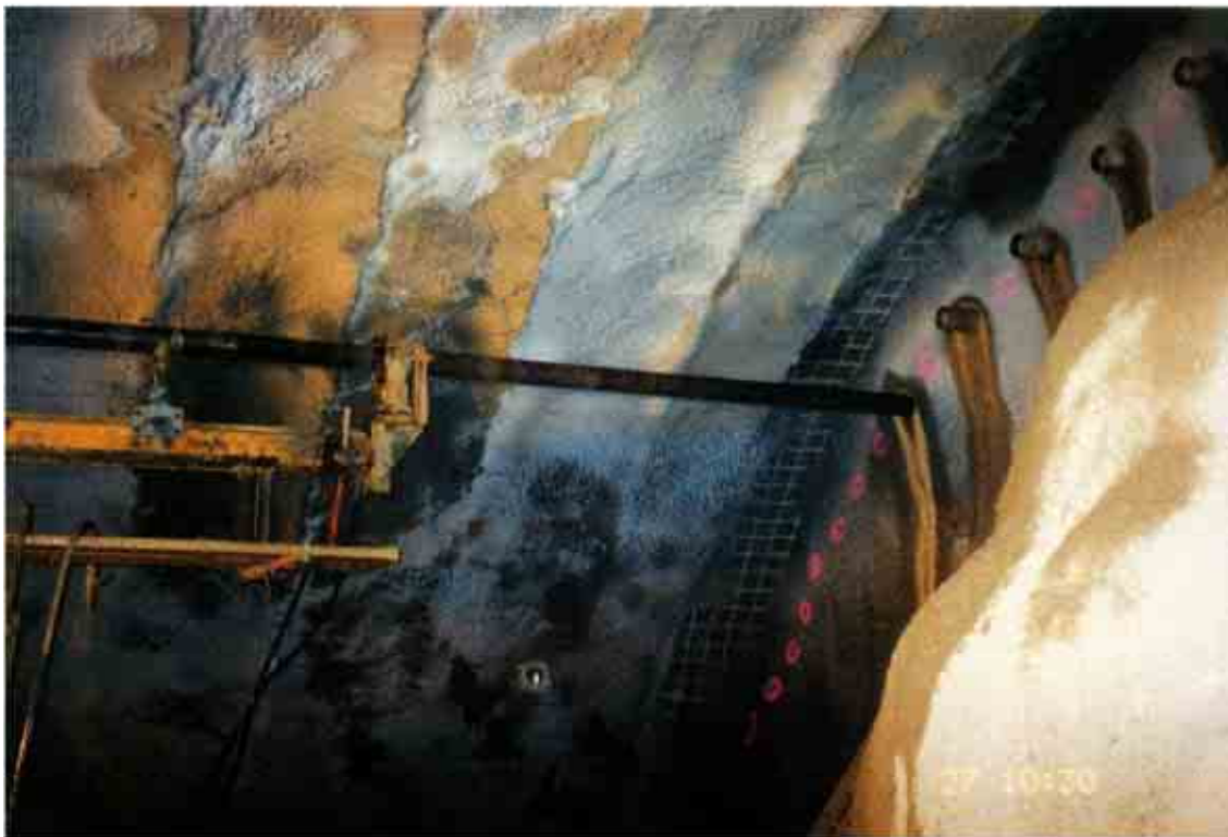
Fig. 2.31: Pipe umbrella in the Dernbach Tunnel (new railway line Cologne - Rhine/Main): a) Pipe umbrella; b) installation of a pipe
