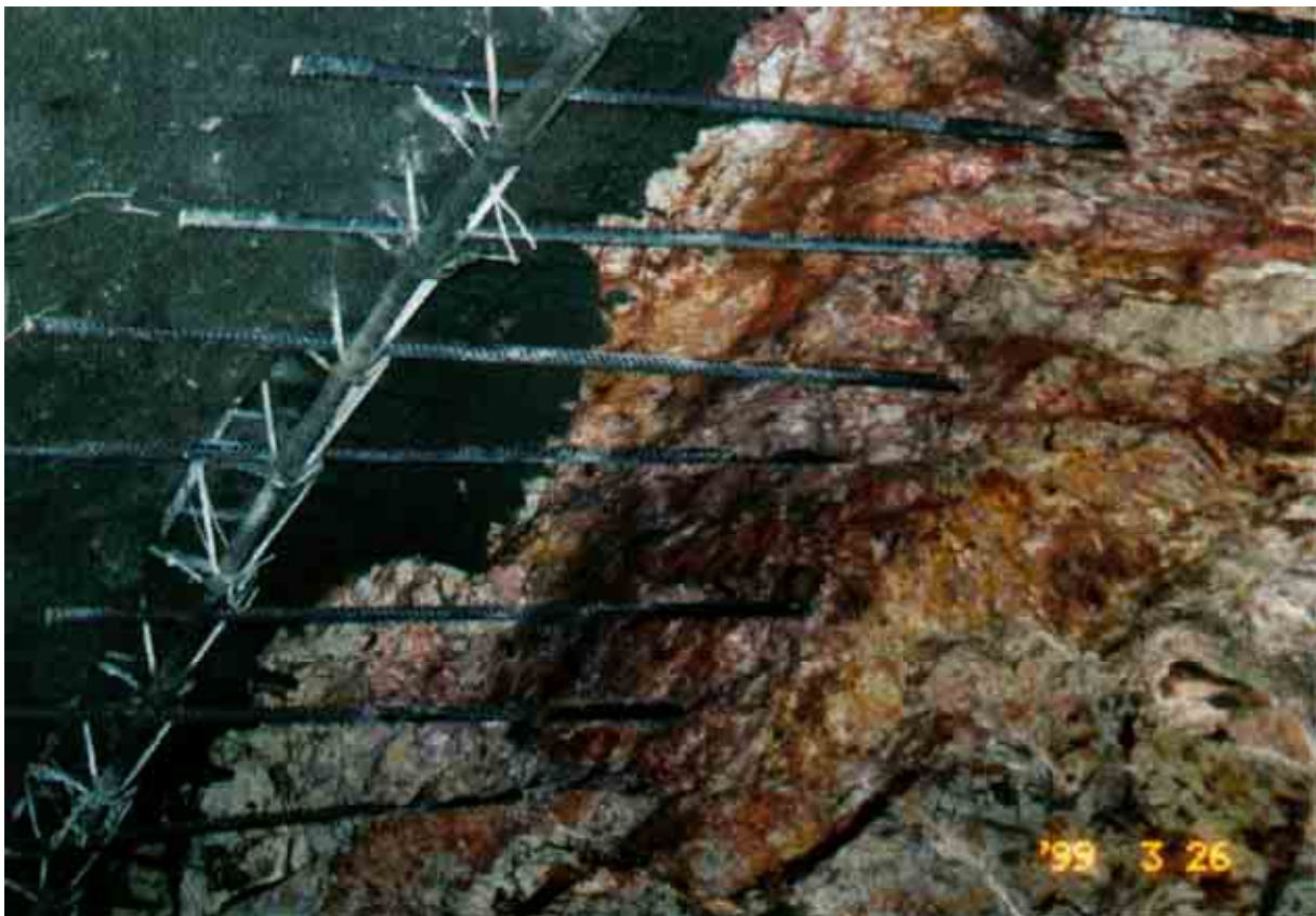
Fig. 2.27: Mortar spiles with lattice girder, blasted free
