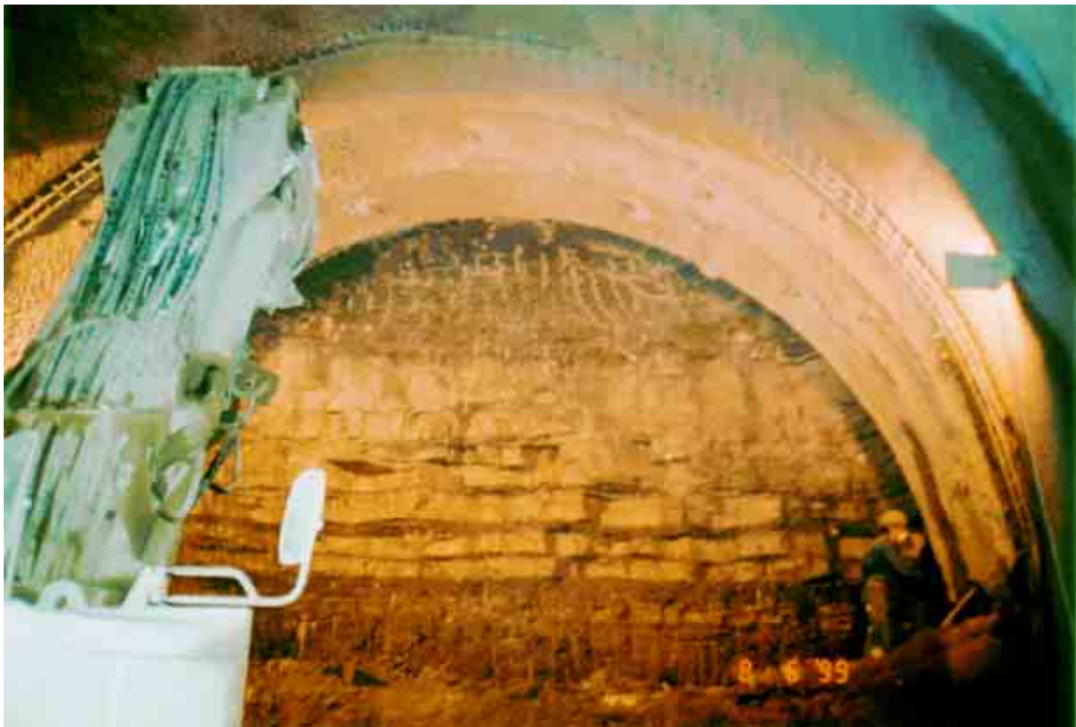
Fig. 6.5: Photograph of the tunnel face showing the transition from the alternating sequence of mudstone and lime-sandstone to the layers consisting predominantly of mudstone
