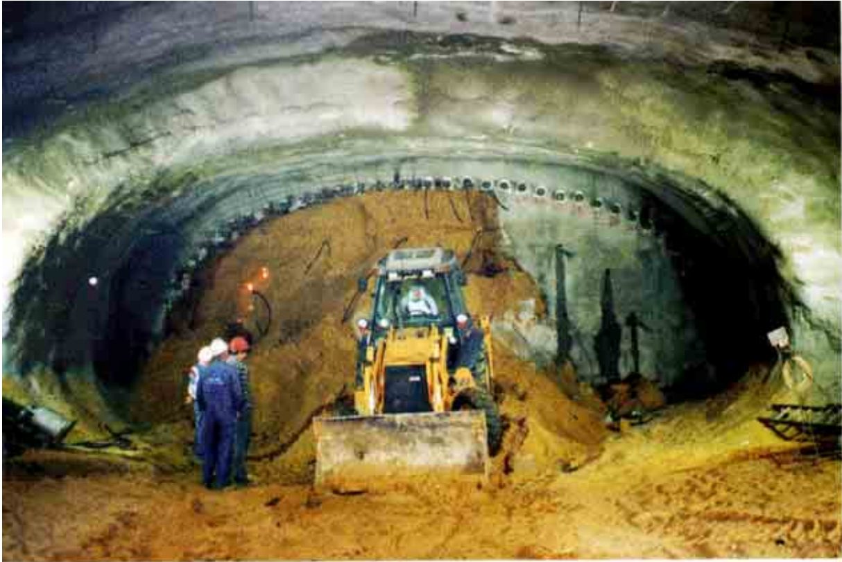
Fig. 4.47: Crown excavation in parts
