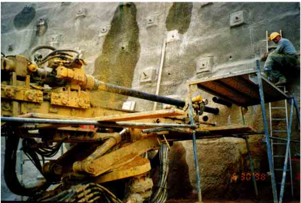
Fig. 2.34: Construction of the pipe umbrella at the starting wall of the Dernbach Tunnel (new railway line Cologne - Rhine/Main)
